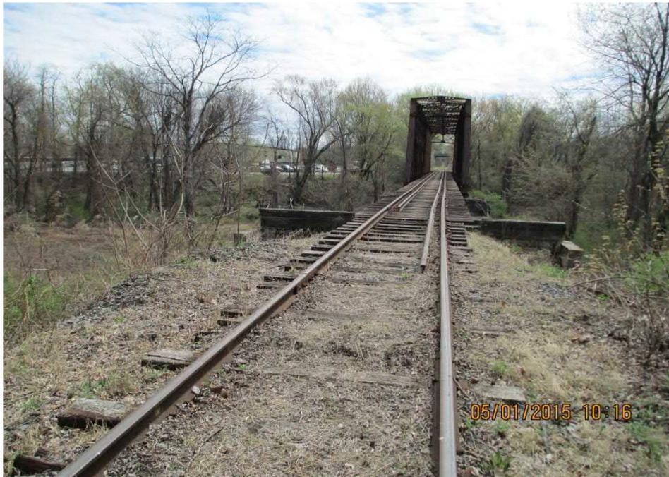
**Looking East at the existing U&D Railroad bridge over the Esopus Creek. The existing structure will be rehabilitated for Alternative 2.**
